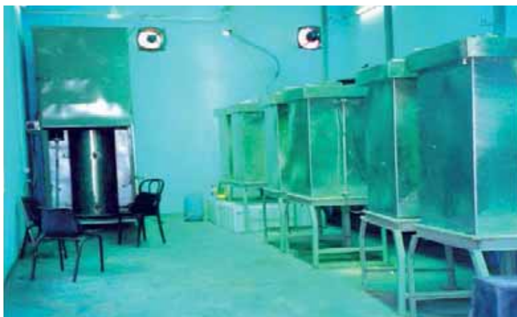
A TEAM plant at Neptha Cracker Unit, IOCL, Panipat, Haryana
