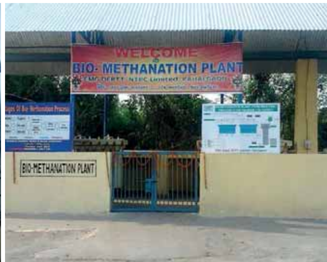
Bio-Methanation Plant, NTPC Ltd, at Kahalgaon, Bihar
