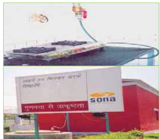
A TEAM plant at Sona, Haryana
